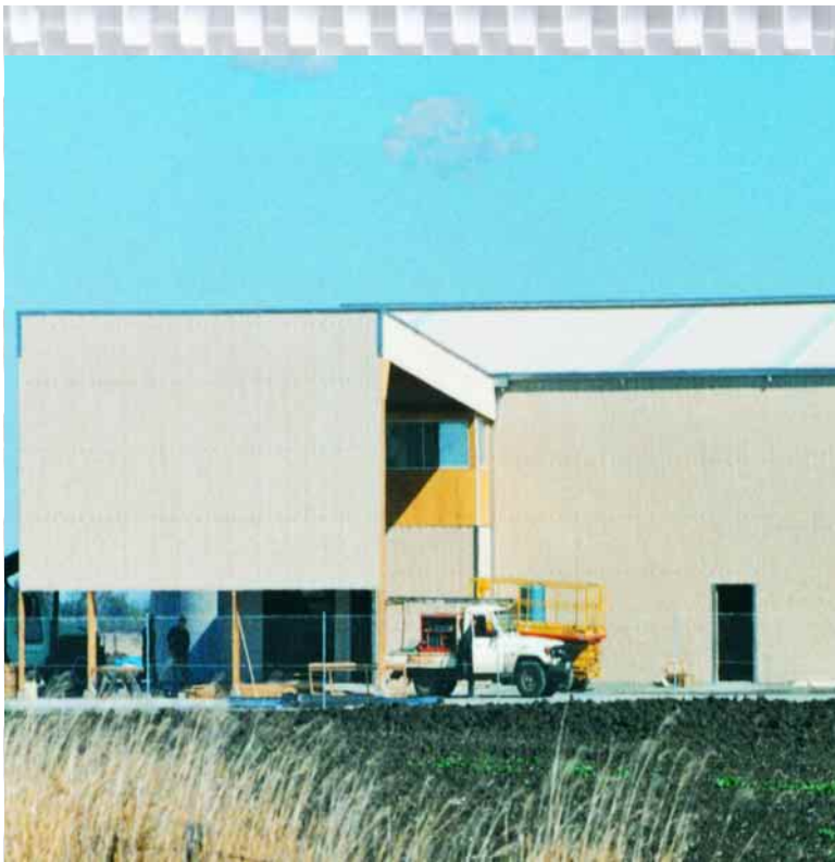
Pivot PFC Warehouse, Brookstead, Qld.
